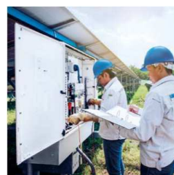
Verify the quality of power from a solar power system
